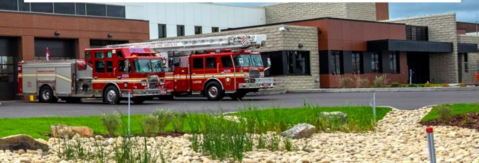
The expanded area of the Protective Services building features equipment bays with room for 18 emergency vehicles.
